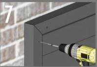
Installing the corner trims is the last part of the project. That makes your project superb finish with Ceta Premium Colour Matched Screws. If placing two trims side by side, these can either be mitered to create a neat angle. Ceta Premium Colour matched screws are available and matched premium range Composite Cladding boards. Corner trims are suitable to use around windows and doors.
