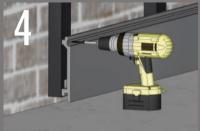
Battens should be attached to the wall at a maximum distance of 450mm apart. The Battens will need to continue to whole length of the area being covered adding in extra Battens at any point where you will need to attach two Cladding Boards end to end Battens should be be fully supported once installed it is important that the surface below the Battens it lat and stable. Remember to install your Battens at a 20-degree angle to the way that you want your Wal Cladding Boards to run.
